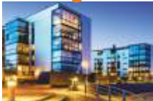
SAUDI ARABIA- RESIDENTIAL BUILDING Merus active filter
