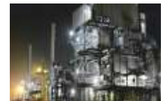
CHINA- WANHUA POYURETHANES CHEMICAL COMPLEX Merus active filter
